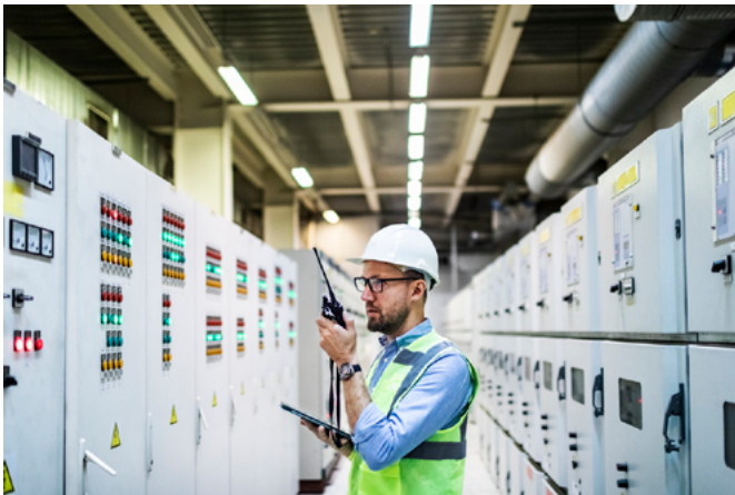
Figure 1: Powering a factory is becoming increasingly challenging
